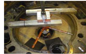
Ball mill housing main bore and flange field restoration
