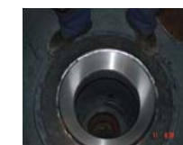
Large Combine valve seats restored in-situ
