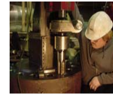
Valve stud hole restoration
